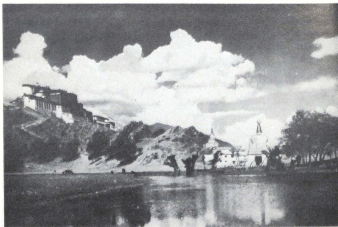
11. The Potala, the Dalai Lama's winter palace, the walls of which were damaged by shelling during the revolt
